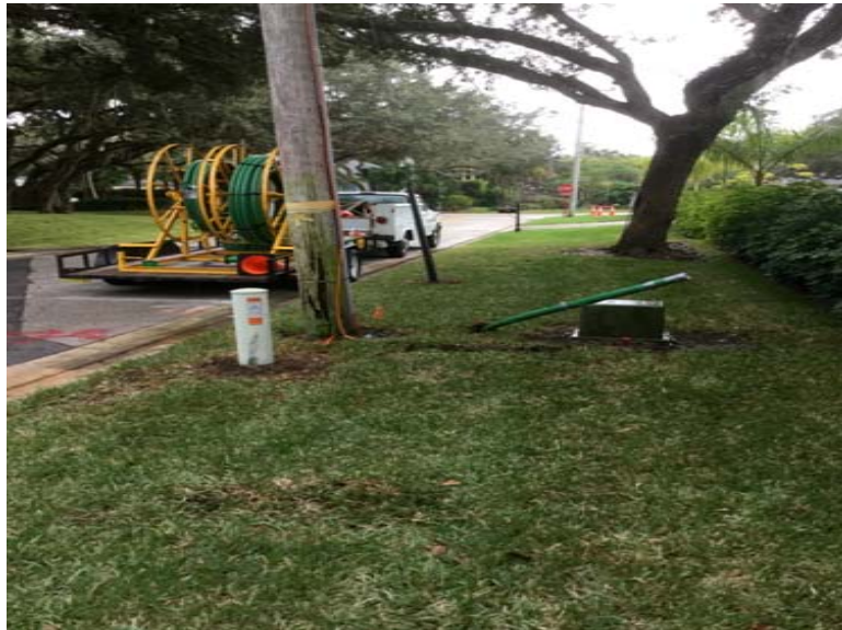
Figure 6. Two-inch main installed.
