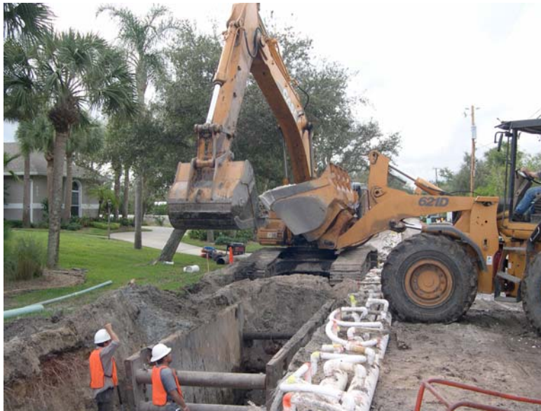
Figure 4. Gravity sewer main excavation.
