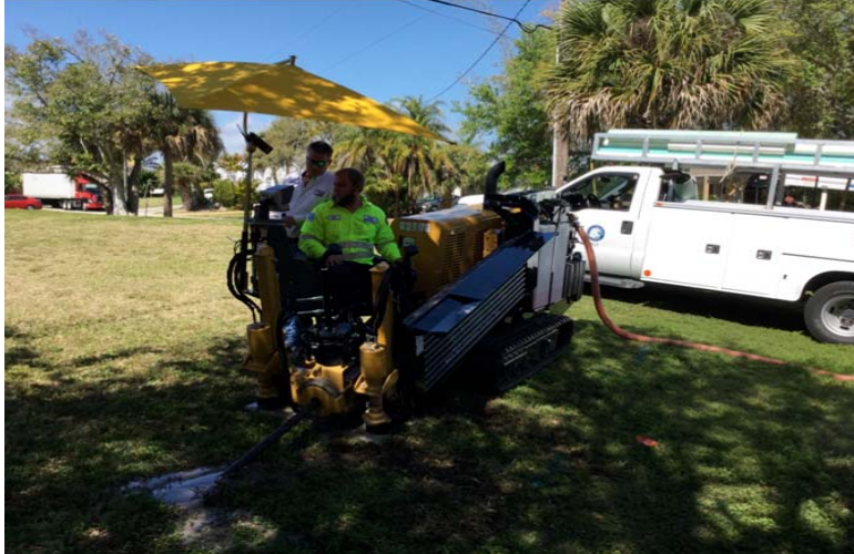
Figure 5. Directional drilling of two-inch main.
