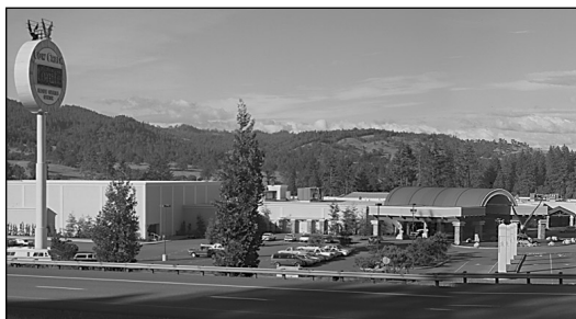
Seven Feathers Hotel & Casino added 30,000 gpd of treatment capacity to its recirculating gravel filter by plumbing six AX100 filters into the existing system.
