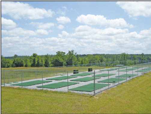
Phase I and Phase II of SAU's West Mobile Wastewater Treatment Plant includes 36 AdvanTex®-AX100 textile treatment units. Two additional phases of similar size are planned. Another 18-pod textile treatment system is under construction in a different location.
