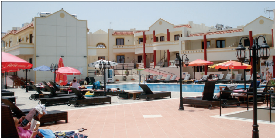
This 5-star Greek resort selected an AdvanTex® media filter, manufactured by Orenco®, to replace its failing wastewater system.
