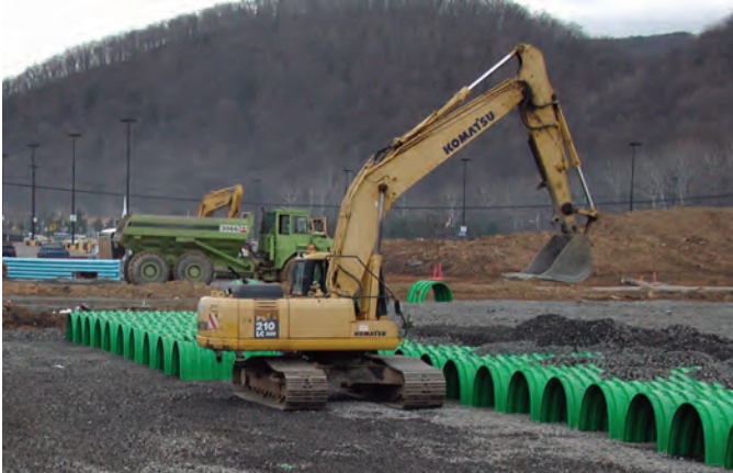
Installing embedment stone around chambers.
