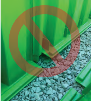
Improper installation. The flange of the chamber is not supported.
