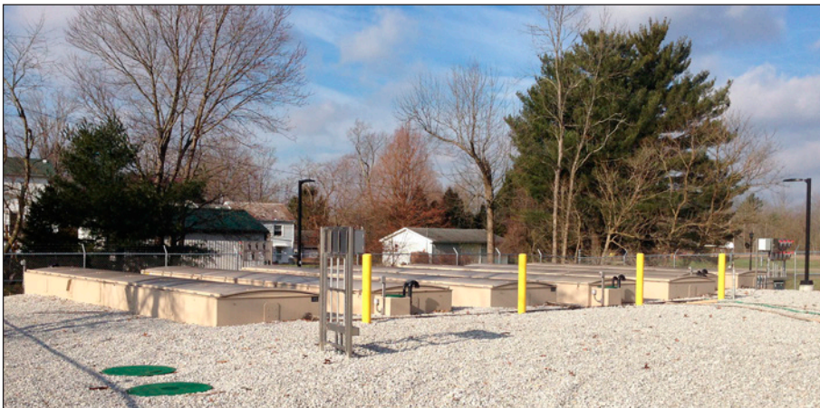
An Orenco Sewer™ collection system, followed by these AdvanTex® AX-Max™ treatment units, was estimated to cost Lore City approximately $1.1 million less than a gravity sewer with a package treatment plant.
