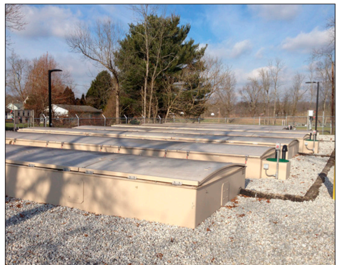
AdvanTex systems use a fixed-film, attached-growth treatment process, an excellent solution for smaller communities like Lore City.
