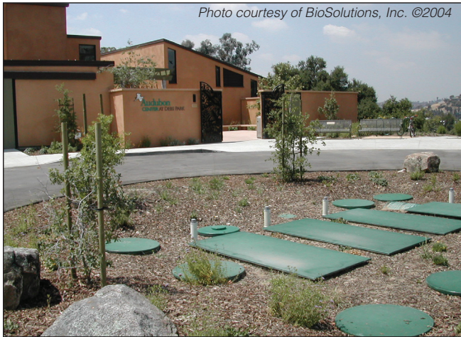
The Audubon Center's AdvanTex Treatment System produces such clear, odorless effluent that it is re-used for irrigation, and, when permitted, will also be re-used for toilet flushing.
