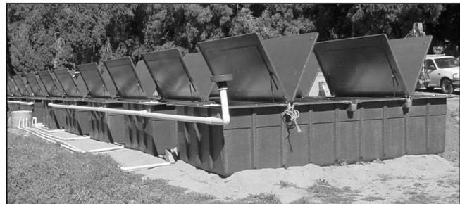
*Design features make it easy to access and service the AX100’s textile filter pods.*
